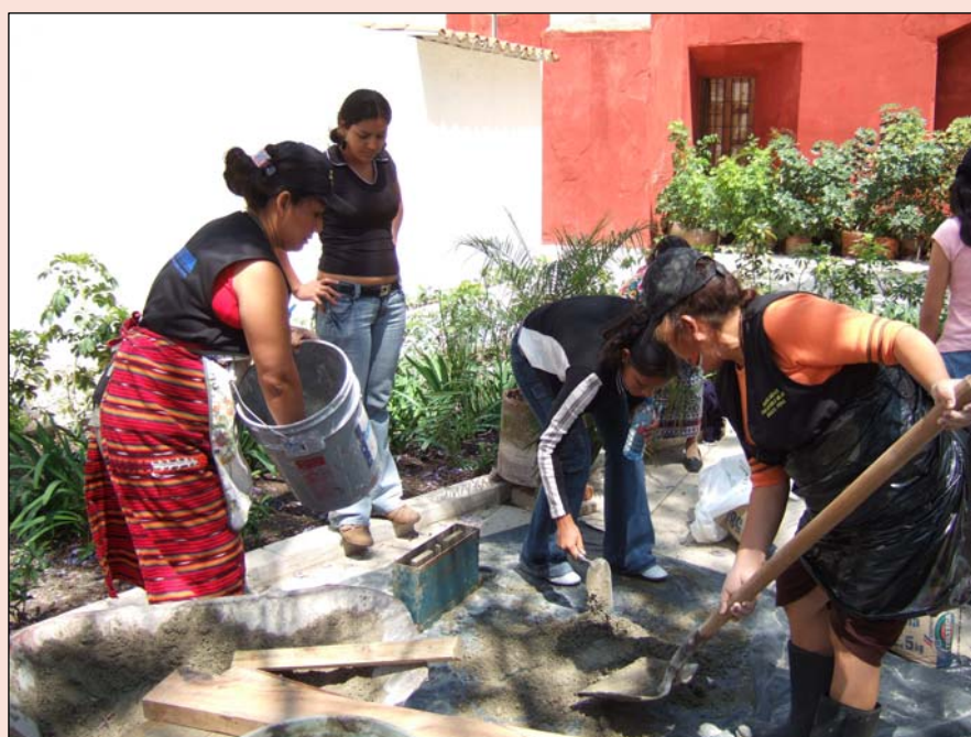
An indigenous women's group builds earthquake-resilient homes, Guatemala, March 2008, IFRC/Provention
